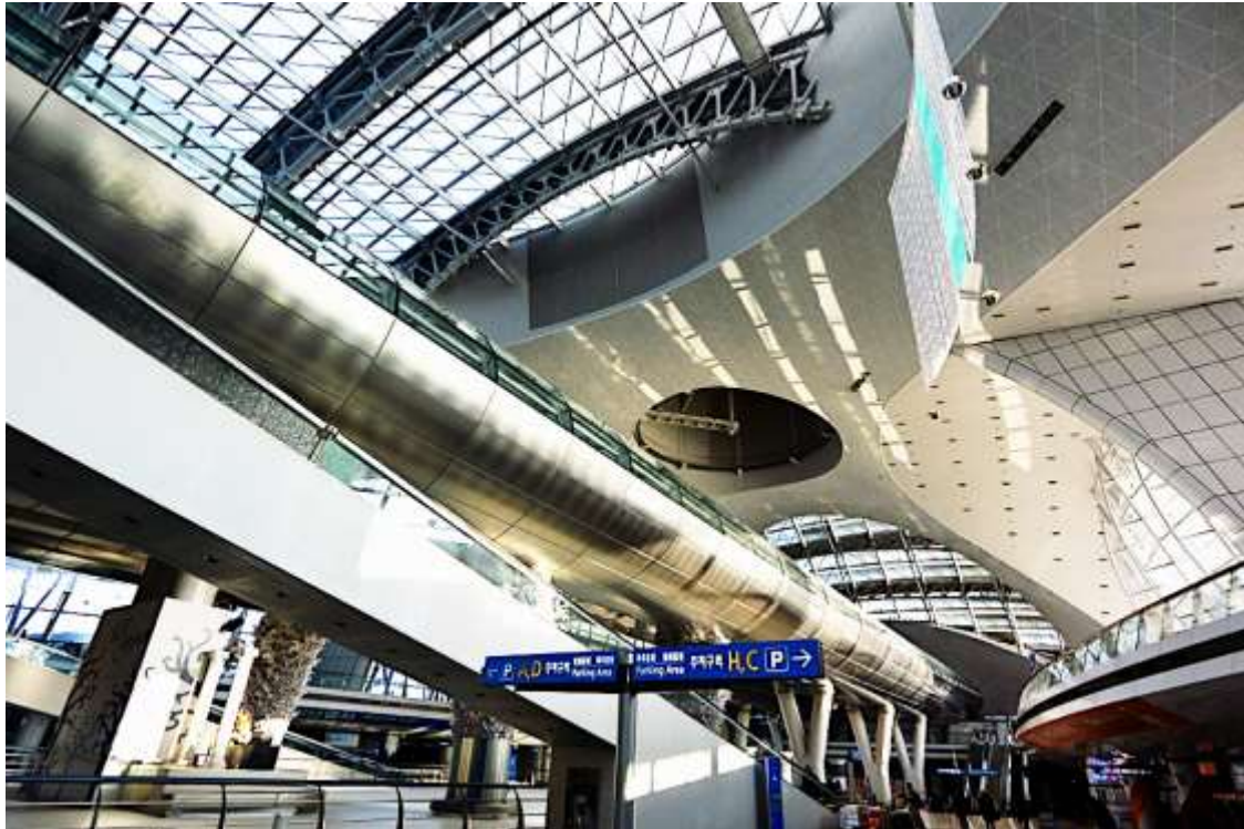
Figura 377. Incheon International Airport.
