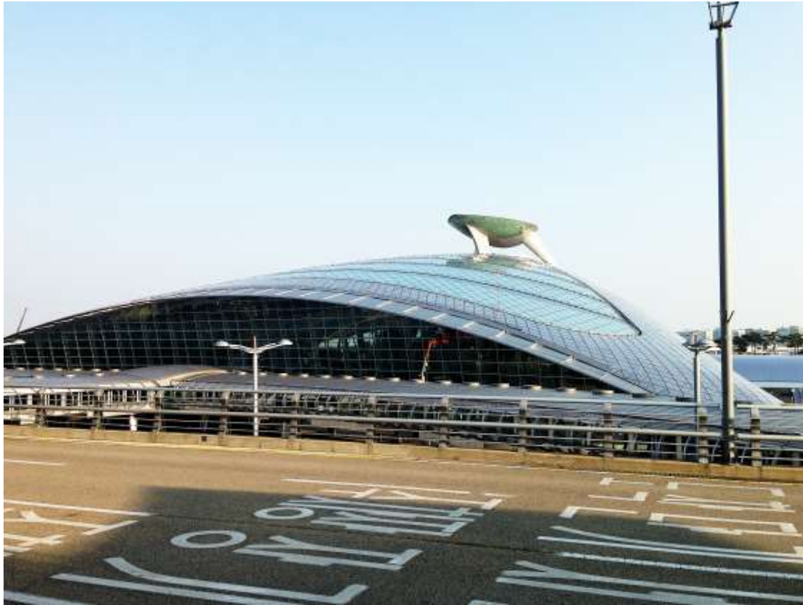
Figura 365. Incheon International Airport.
