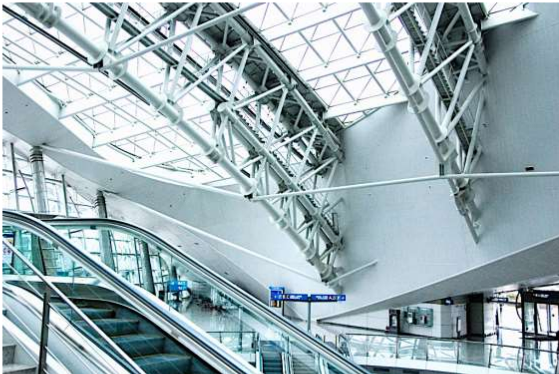
Figura 368. Incheon International Airport.
