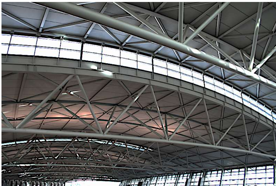
Figura 382. Incheon International Airport.
