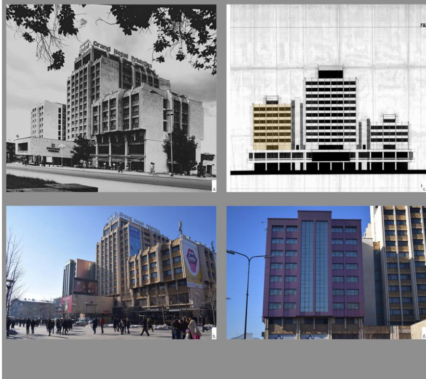
Figure 9. Hotel Grand, B. Fehmiu, M. Jevremovič and D.Kovačević, Pristina, 1978; Comprehension of the initial state (a) with the interventions after the latest renovation. Part of the facade that has been coated with contemporary materials (c). Detail of the current state of the façade (d). © Credits: a, c: Gjinolli, Ilir. and Kabashi. Lulzim. Kosovo Modern: An Architectural Primer. Prishtina: National Gallery of Kosovo, 2015; b,d: authors
