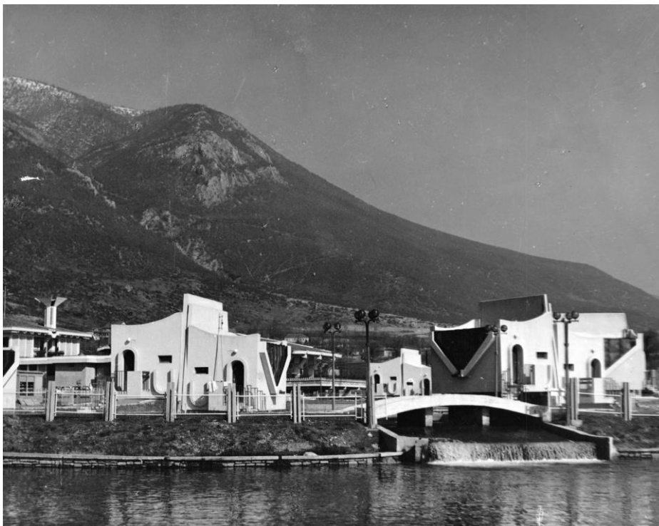
Figure 6. Motel "Trofta", Q.Beqiri, Istog, 1979. © Credits: Gjinolli, Ilir. and Kabashi. Lulzim. Kosovo Modern: An Architectural Primer. Prishtina: National Gallery of Kosovo, 2015
