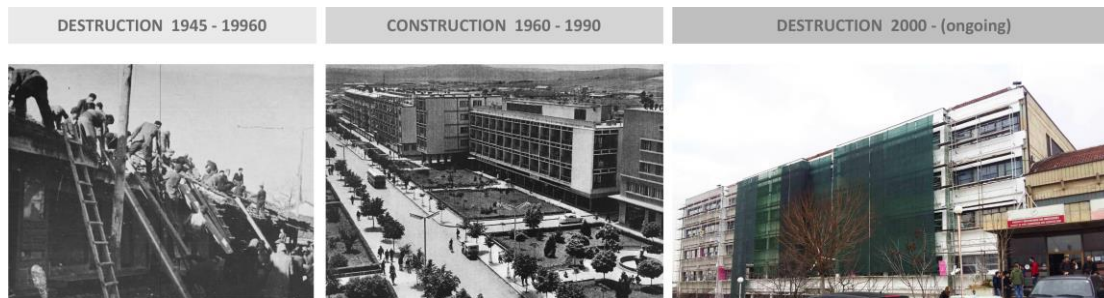
Figure 11. The process of the evolution of Kosovo Modernism a. destruction of the Old Market (Çarshia) in Pristina; b. construction of the city center of Pristina; c. renovation of the Technical Faculty in Pristina, designed by Edvard Ravnikar. © Credits: a. Cultural Heritage Without Borders. Heritage of Pristina – Remained Heritage of Pristina. Pristina: Prograf, 2008; b. Časopisa “Revija”. Gradovi Jugoslavije, Grafički Zavod Hrvatske, 1965, c. authors
