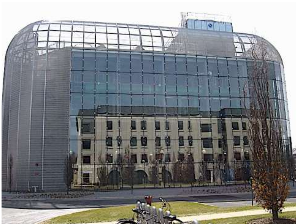
Figura 216. University of Chicago South Campus Chiller Plant (Burimi): angwe23, 2009. (Flickr). Creative Commons–NoDerivs 2.0 Generic
