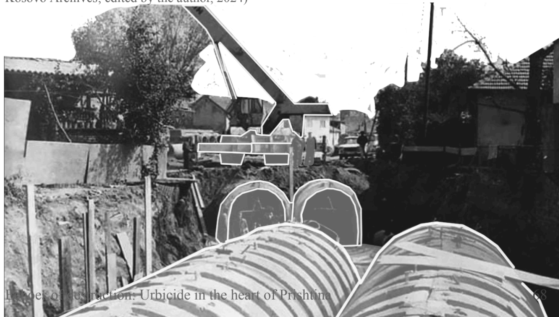
Fig. 40 The Prishtina River as it sinks under concrete and becomes a man-made sewage system (Source: Kosovo Archives; edited by the author, 2024)
