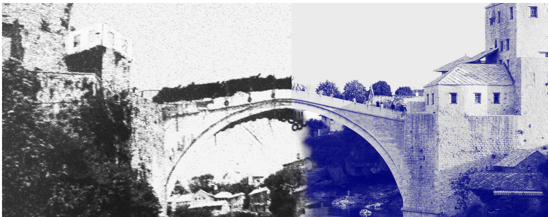
Fig.11 Mostar Bridge, yesterday and today. (Source: edited by the author)
