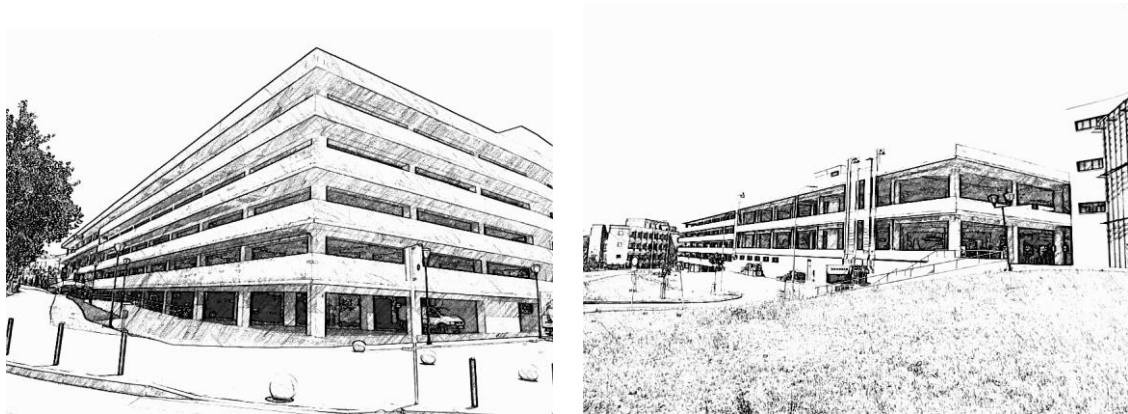
Figure 5. First City Public Parking Garage, Prishtina. [Source: Authors, 2016]
